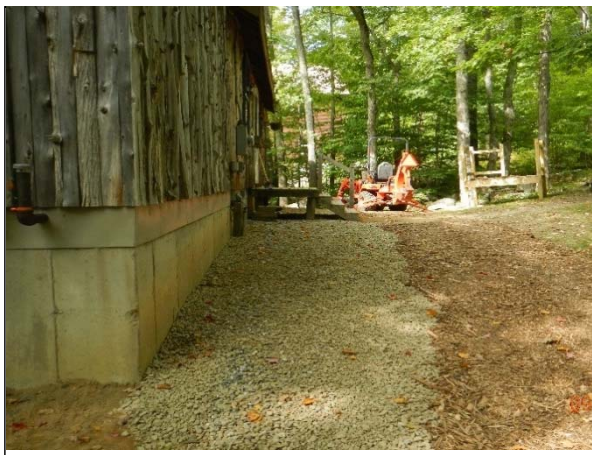
Drip-line infiltration trench installation
